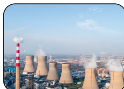
RENEWABLE ENERGY SYSTEM
